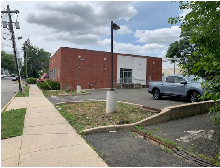
Rear of Building/Parking Lot
