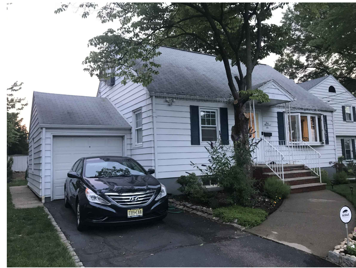
VIEW OF EXISTING HOUSE
